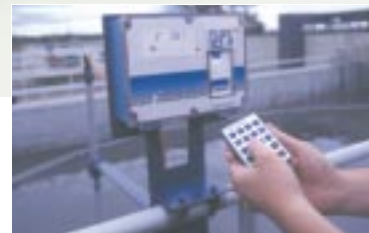
Setting up the DPS 300 on-site with the infrared, handheld programmer. Electronics are not exposed.
