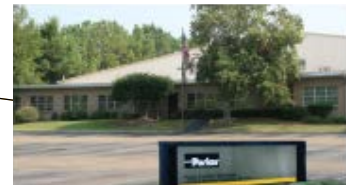
Fluid Control Division Facility, Madison, MS.
