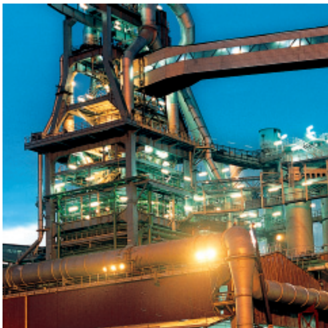
Industrial application: Refinery
